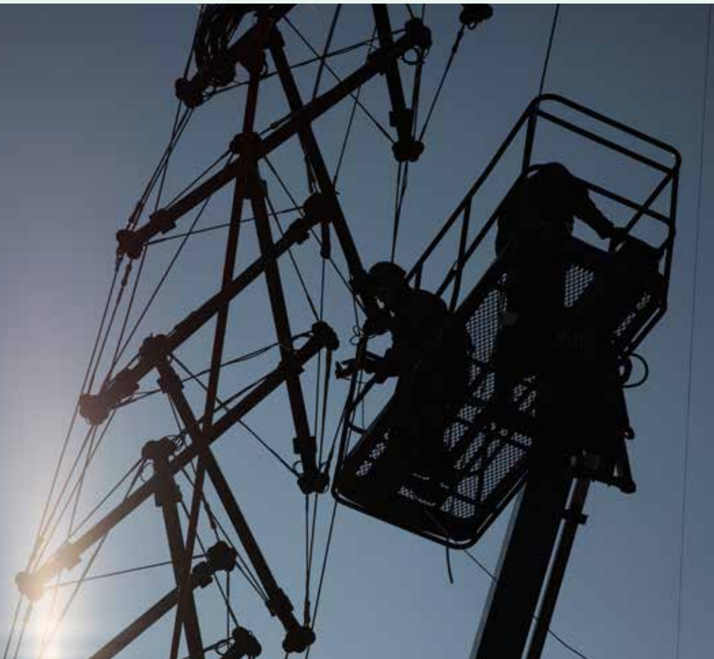
↑ Inox-Litze Toron Inox Stainless steel strand 1 x 19 E = 1,4 - 1,7 · 10 5 N/mm 2
